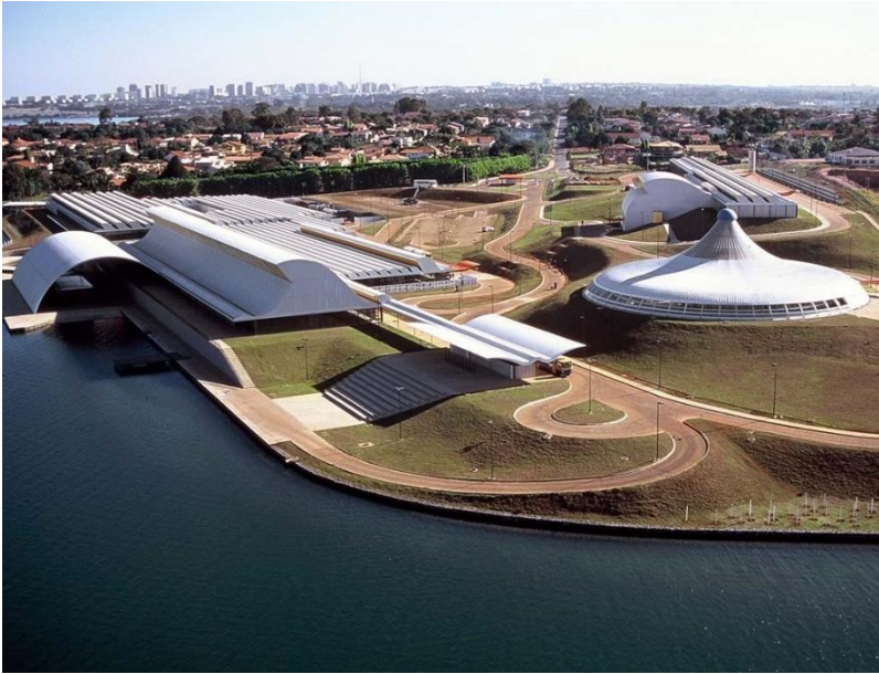
Overview of the Sarah Kubitchek rehabilitation center and educational facilities at Lago Norte in Brasilia (1997-2003)
