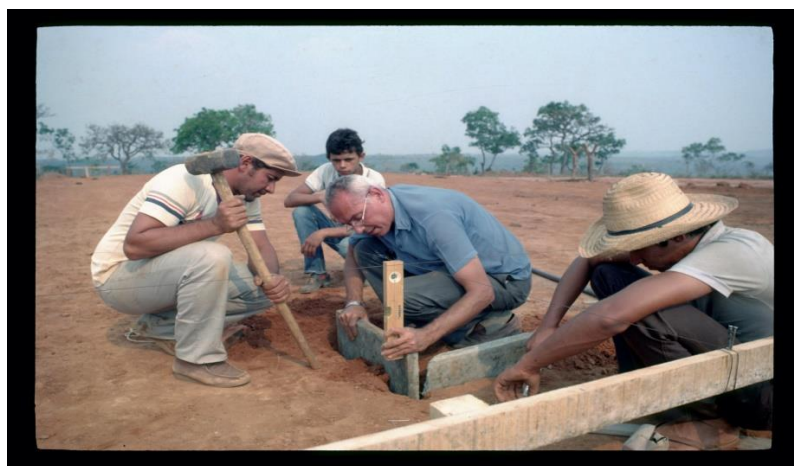
Abadiania experimental school system: Lele teaching the workers how to prepare the ground for putting up a column
