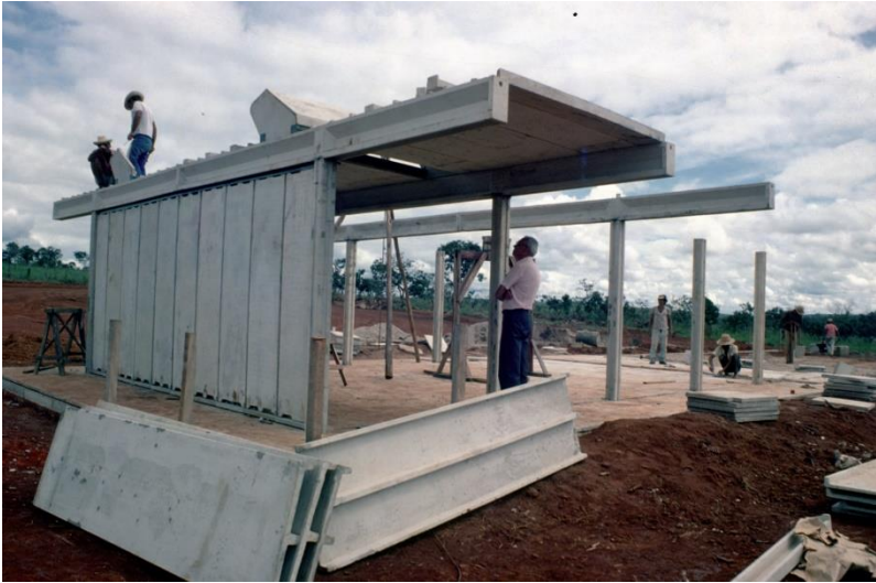
The placing of the modular wall-elements
