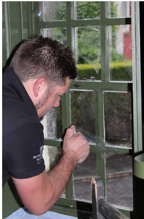
FIG. 4 - Removing UV film for an installation. © National Trust for Scotland.
