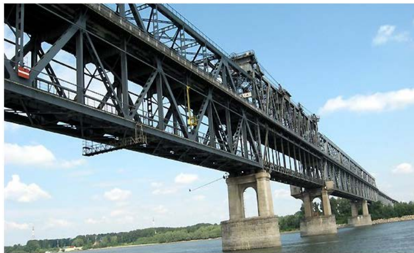
Fig. 4. The Danube Bridge, the town of Ruse.
