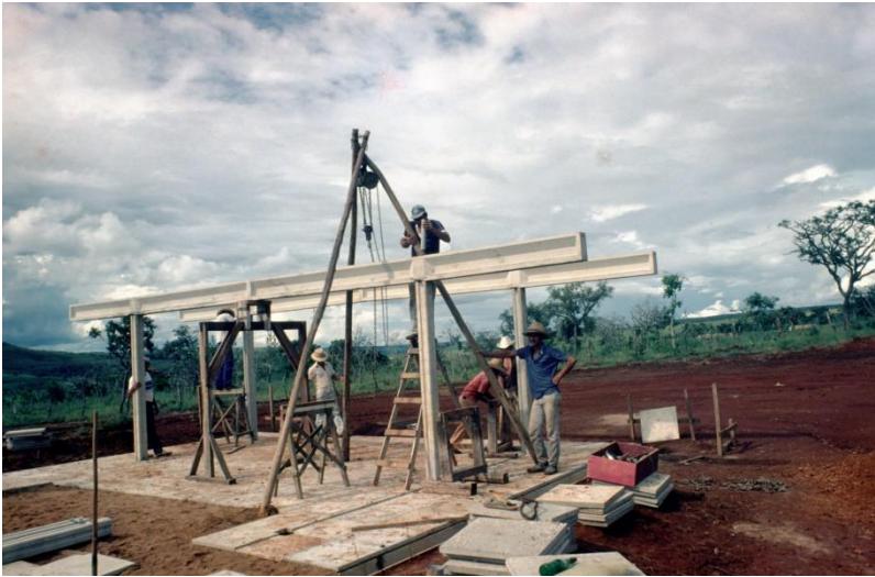
Lele assisting the assembling of the gutter-beams to the columns
