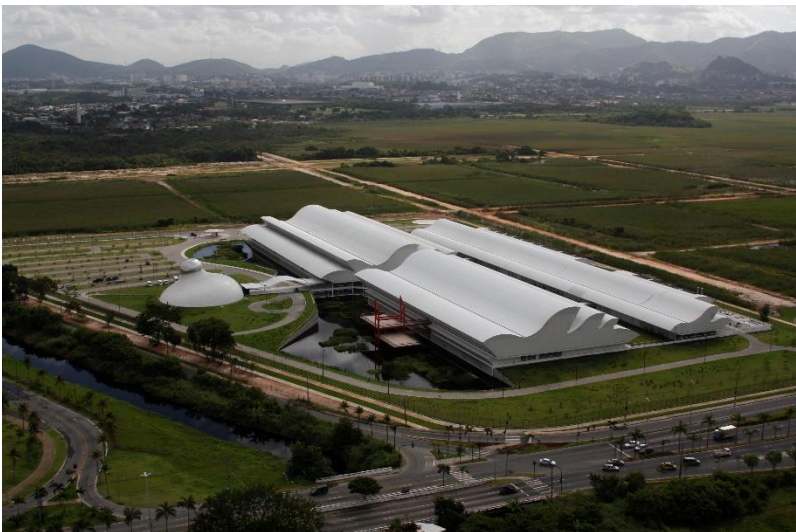
Overview of the Sara Kubitchek hospital in Rio de Janeiro (1999-2010)
