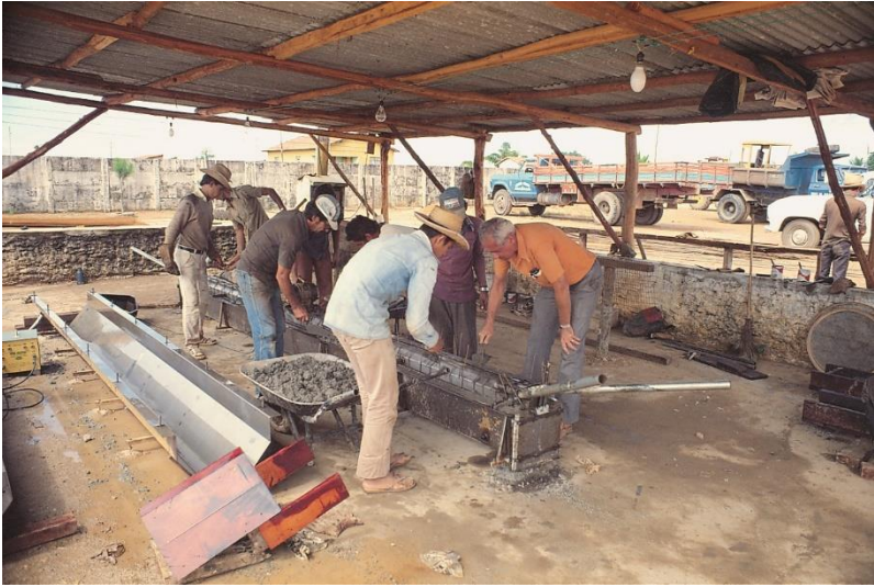
The metal molds in use at the workshop in Abadiana
