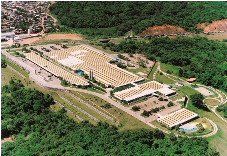
Overview of the Sarah Kubitschek hospital and revalidation Centre in Salvador (1991-2001)
