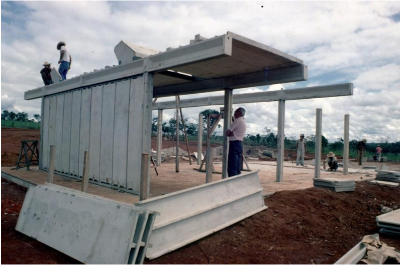
The placing of the modular wall-elements
