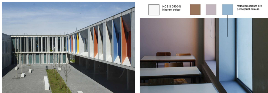
FIG. 11 - Reflected colours in the classroom. Braancamp Freire School, Lisbon. Colour Consultant: João Pernão.
