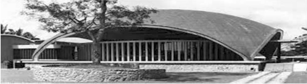
Plate 4: Sultan Bello dining Hall, University College, Ibadan. The hall comprised a shallow reinforced-concrete dome rising from slender elliptical ribs over semi enclosed walls.
