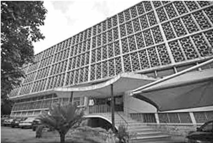
Plate 3a: The approach view of Kenneth Dike Library, University of Ibadan, Ibadan. The library was designed with access corridors on each bank and interior shutters to protect books from storm damage. The library was a five – story building.
