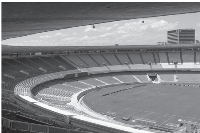
Fig. 3. The Maracãna Stadium before 2014.
