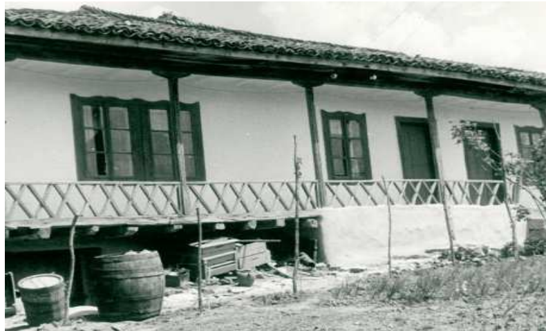
2. Old traditional house in Dobrudja agricultural area - there is no stone.
