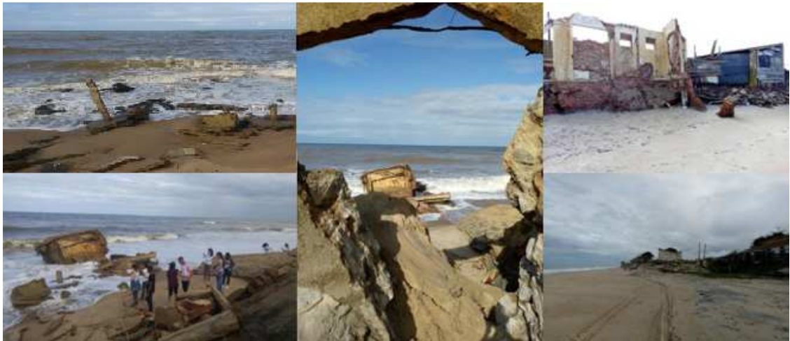
Figure 1 – Damage caused by marine transgression in Atafona, RJ, Brazil (Caetano, 2018).
