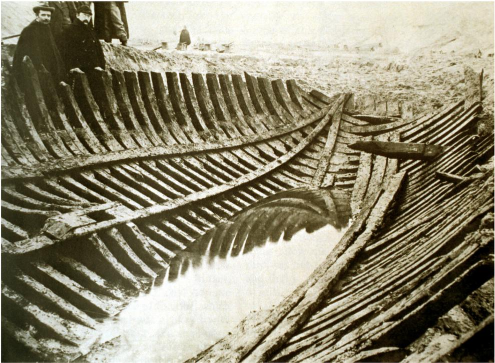
Fig. 2.21. View of the hull bottom of the *Contarina 1* shipwreck in the River Po delta in 1898
