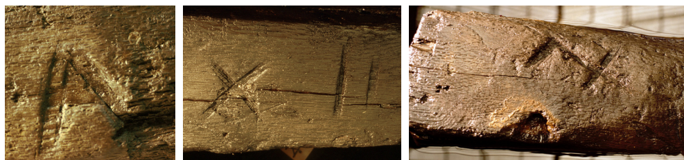
Figs. 2.24a to 2.24c. Latin numeric marks (V, XII and XV) engraved by excision in the preserved frames 5, 12 and 15, as indicators of position in the architectural sequence
